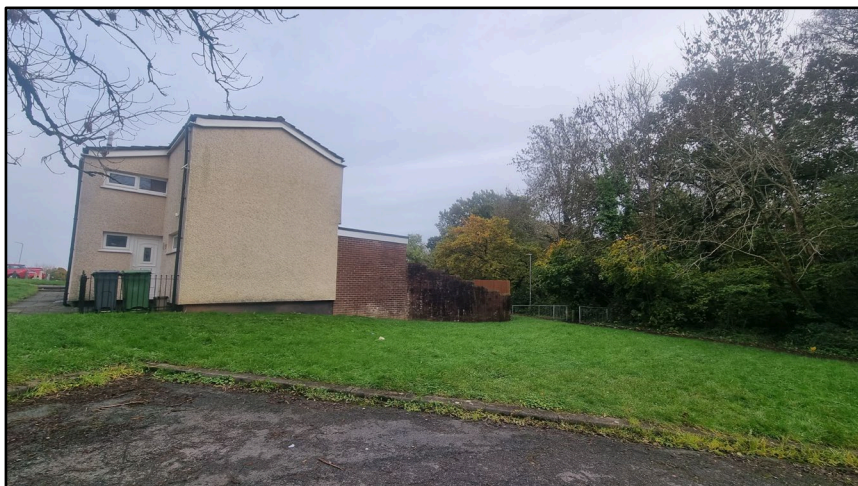
Figure 14: Western Elevation (204 Brynfedw)
