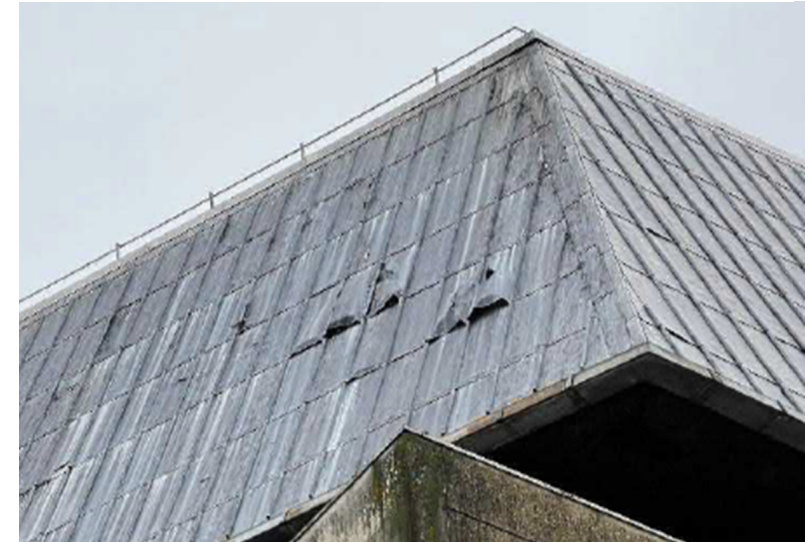
Lead faced Mansard Vertical Roof
