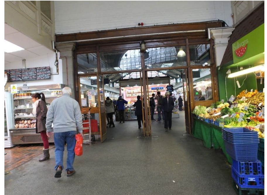
New purpose made Welsh language signage is proposed to be installed above the inner door. Inner doors to be replaced. Current stall installations conceal many of the buildings fine features eg pilasters
