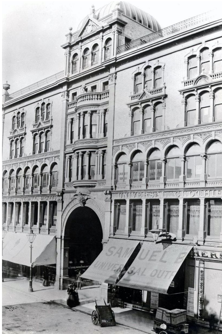
St Mary Street Entrance circa 1895 and 1975
